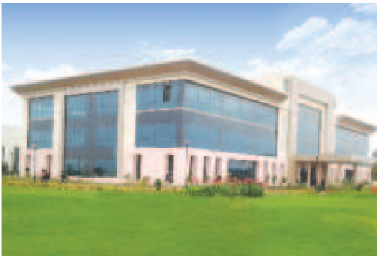
Switchgear Factory, Vadodara
