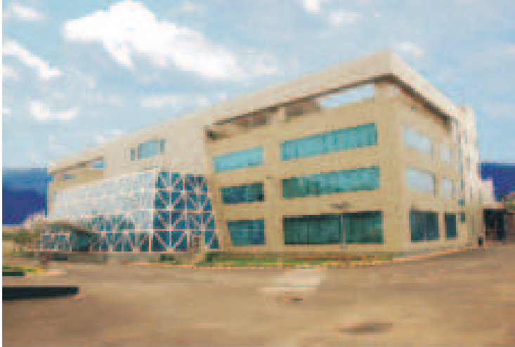
Switchgear Factory, Navi Mumbai
