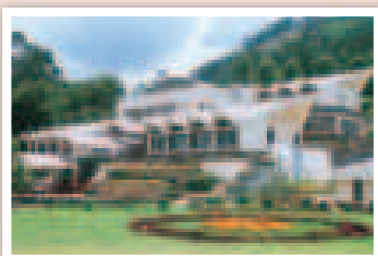
Coonoor L&T Electrical & Automation Training Centre Ooty-Coonoor Main Road Yellanahalli P.O., The Nilgiris - 643 243 Tel. : 0423 251 7107 E-mail: stc-coonoor@Lntebg.com
