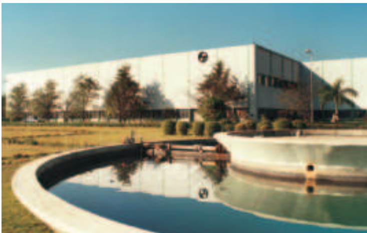
Switchgear Factory, Ahmednagar
