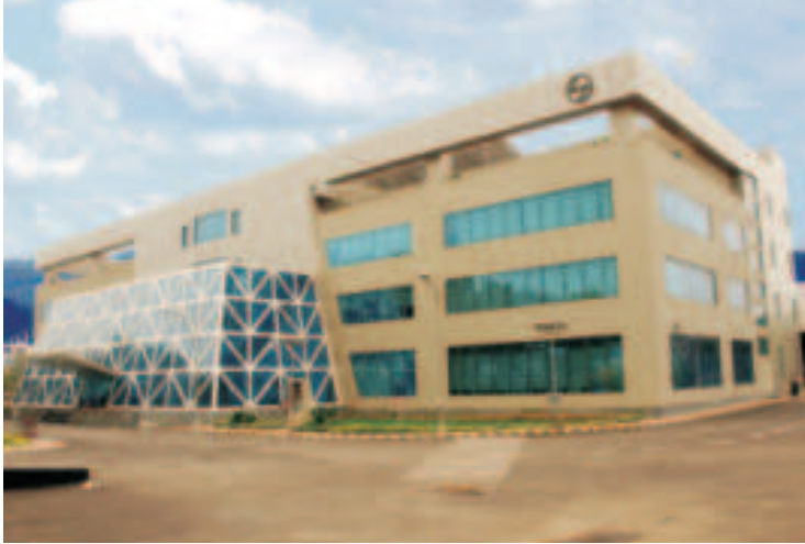
Switchgear Factory, Navi Mumbai
