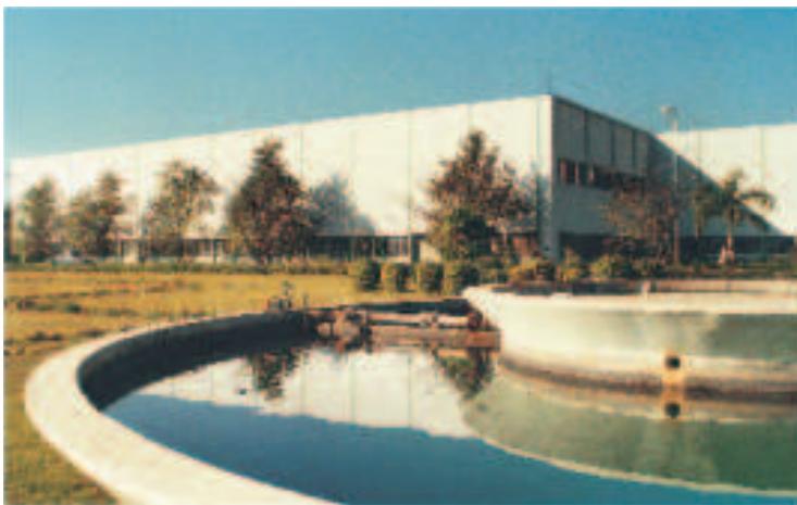
Switchgear Factory, Ahmednagar
