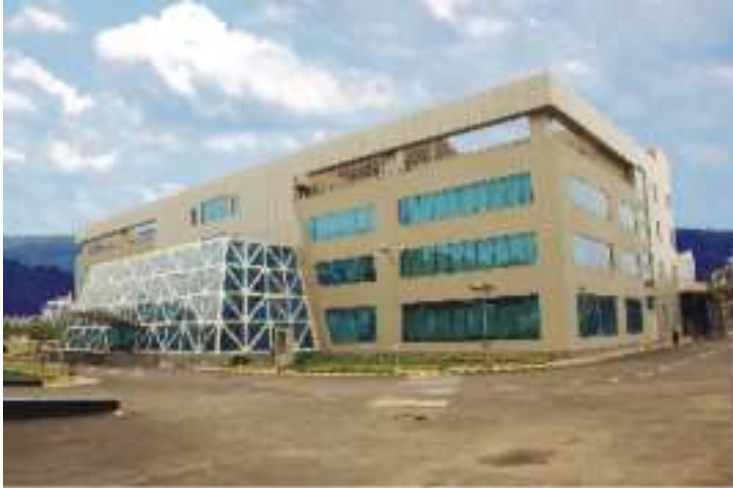
Switchgear Factory, Navi Mumbai
