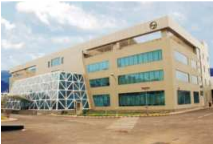
Switchgear Factory, Navi Mumbai
