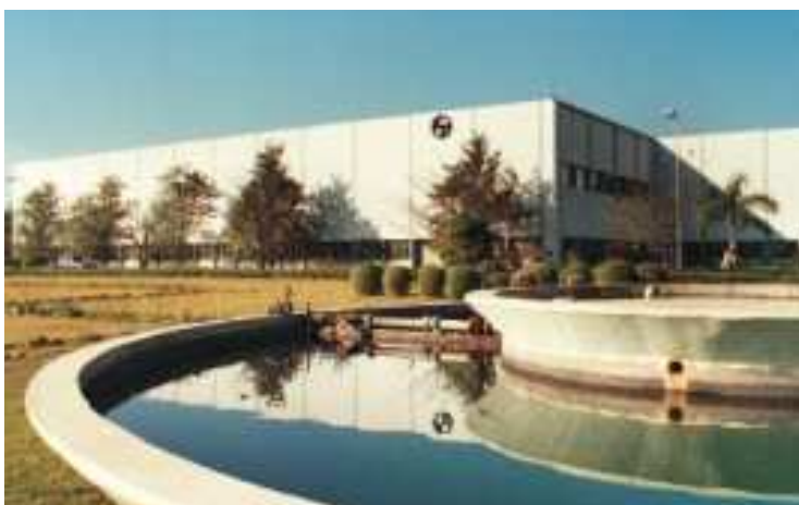
Switchgear Factory, Ahmednagar
