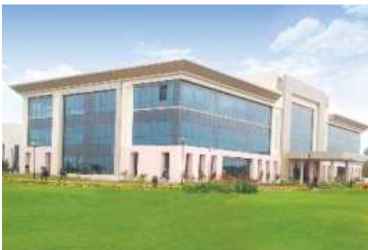
Switchgear Factory, Vadodara
